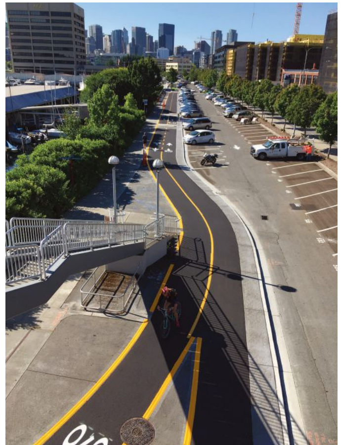
Before (left) and after (right) images of the parking lot along Westlake Avenue that was modified to incorporate a cycle track while preserving 90-percent of the parking.
