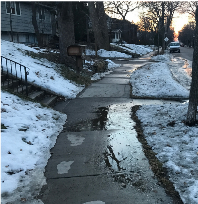
Figure 15. This sidewalk is lower than the adjacent yards, resulting in pools of standing water in the pathway of pedestrians.
