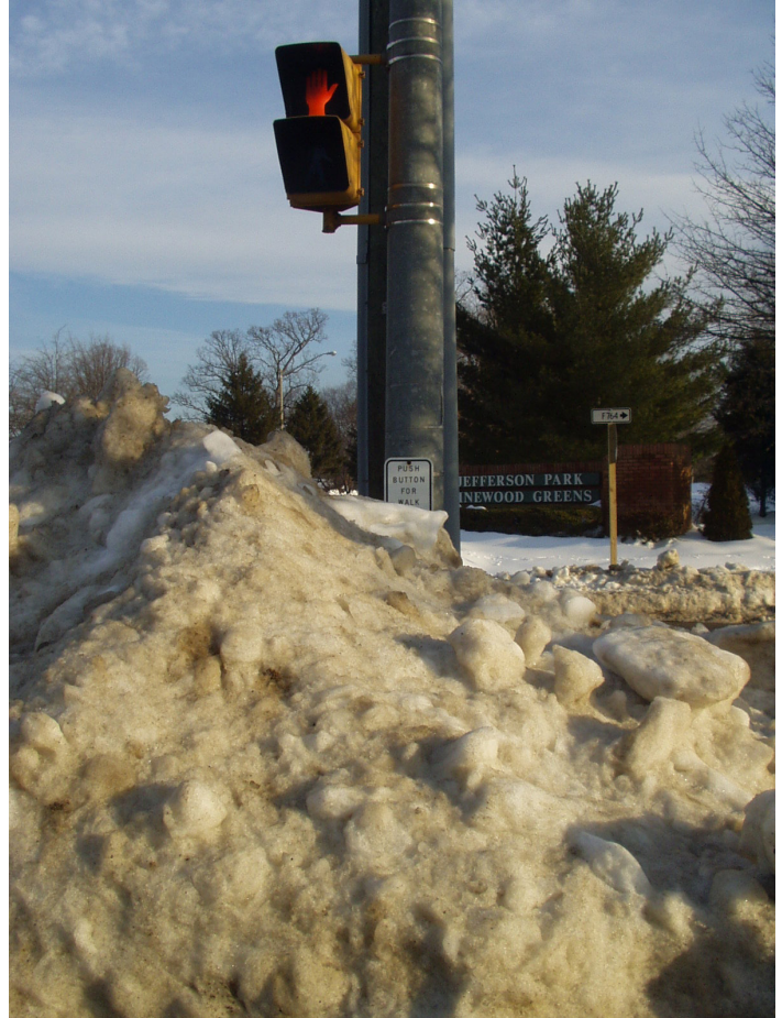
Figure 14. Snow piled in front of pedestrian push buttons prevents people with disabilities from activating the signal.
