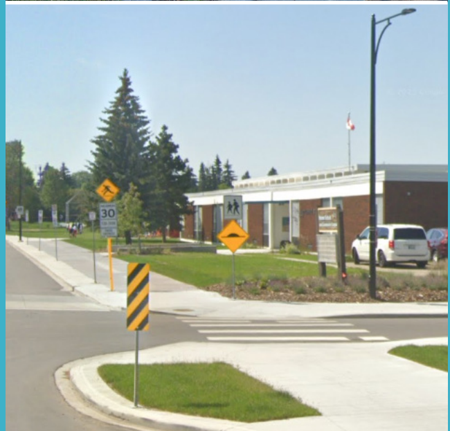
Figure 12: Reflective vertical elements can be used to alert snowplow operators to the presence of curb extensions. Top: U-channel post with reflector in Portland, OR; Bottom: Hazard marker in Edmonton, AB. Photo credit: Google Street View
